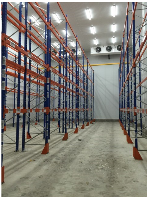
Figure 21: Racking system in place under newly-constructed ammonia-based cold storage warehouse
